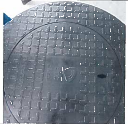
VISUAL INSPECTION (DN-1000 mm)
