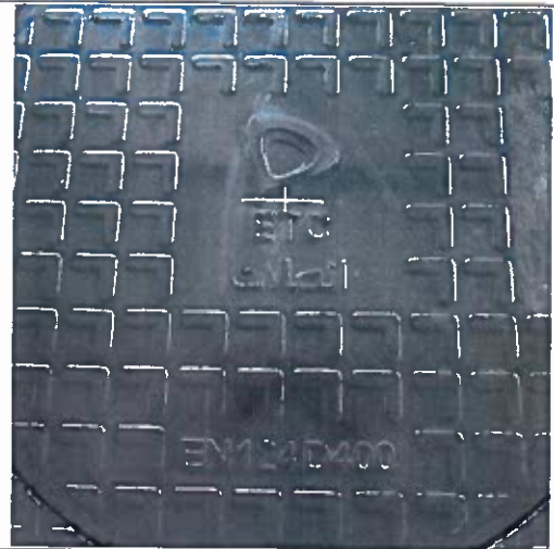
VISUAL INSPECTION (DN-1000 mm)
