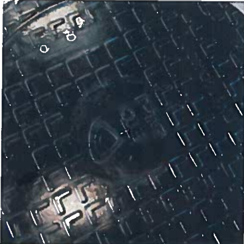
VISUAL INSPECTION (DN-800 mm)
