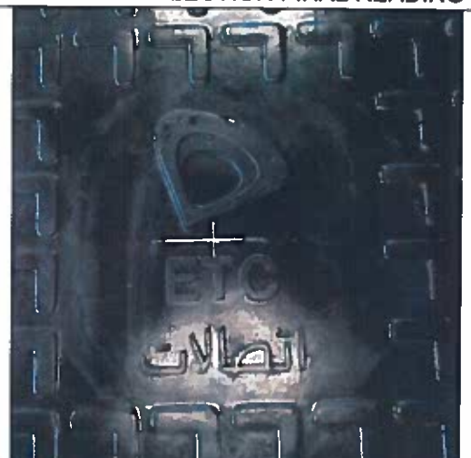
VISUAL INSPECTION (DN-1000 mm)
