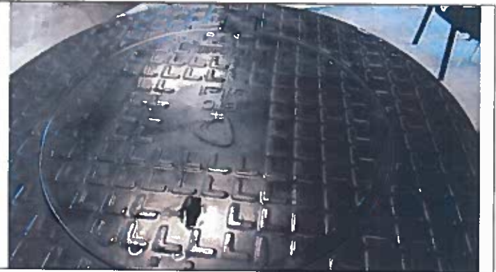
VISUAL INSPECTION (DN-1000 mm)
