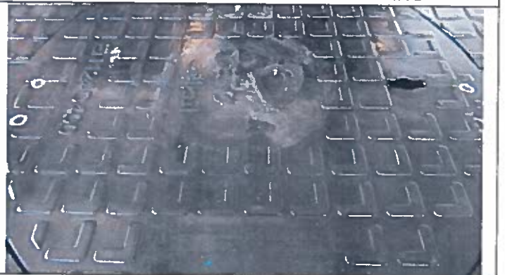
VISUAL INSPECTION (1200 x 800 mm)
